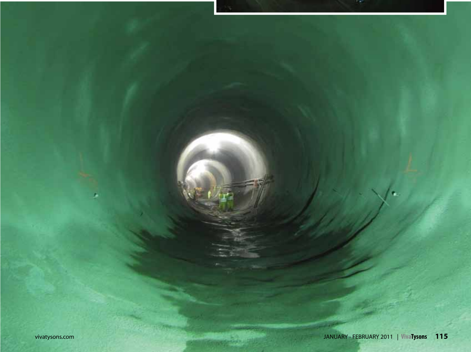
Above: The tunnel entrance at the construction staging area as they travel under International Drive toward Route 7. Below: An eerie green glow from the tunnel walls from a fresh coat of water-proofing that was sprayed on the interior concrete surface as seen to the right.
