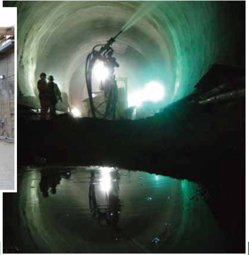
Above: The tunnel entrance at the construction staging area as they travel under International Drive toward Route 7. Below: An eerie green glow from the tunnel walls from a fresh coat of water-proofing that was sprayed on the interior concrete surface as seen to the right.
