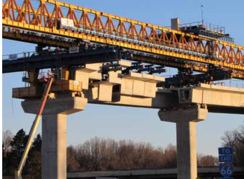
Above: Concrete segments of the spans are lifted and set in place below the horizontal crane crossing Route 123 at I-66.
