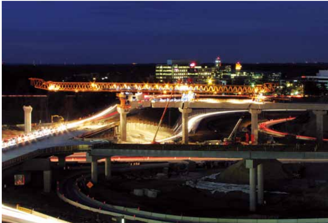
Above: A dramatic night shot of the crane crossing the Westpark Drive Bridge over Route 123. Below: The third crane is assembled that will install the spans across the Beltway.
