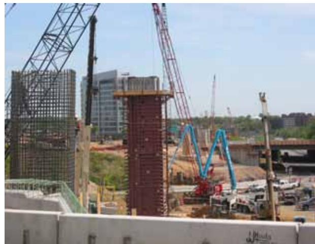
Pier construction is moving fast. This view looking from the Westpark Bridge toward Capital One along northbound 123. These piers will hold up the rail as it crosses over the Beltway. The tremendous amount of structural steel rebar can be seen here before the piers have forms placed around them for the concrete to be poured.
