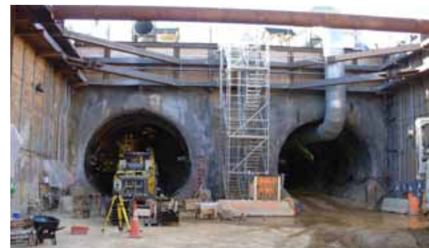
This view of the tunnels from the construction headquarters at International Drive and Route 123 shows the sprayed grey shotcrete around the openings.
